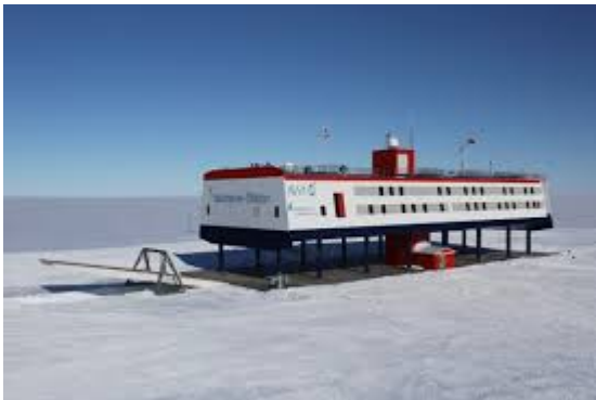
Neumayer III Station
